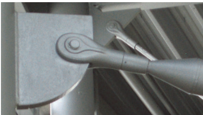
Compression system connected to a welded plate
