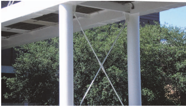
Cross-bracing with a cross coupler
