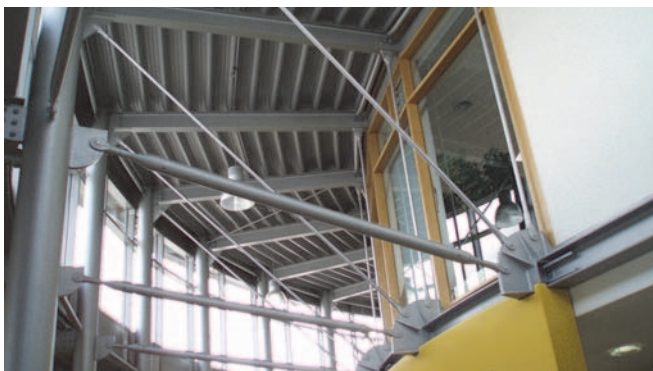
Bracing between an exterior steel column and an interior steel beam
